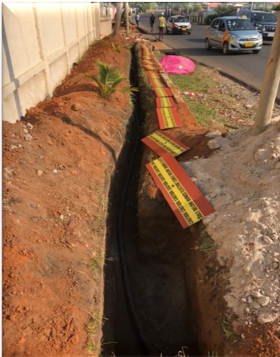
Laying of Under Ground Cable at SS Omane Street – MiDA Project (Kaneshie District)
