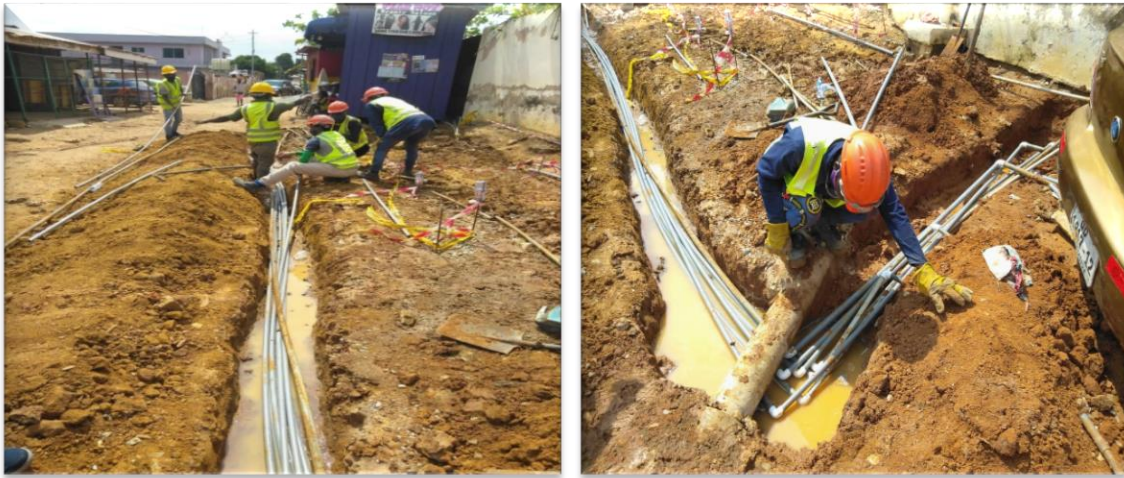
Diversion of pipes and preparing the grounds for GMT Substation Foundation works at Abeka Market down – MiDA Project (Kaneshie District)
