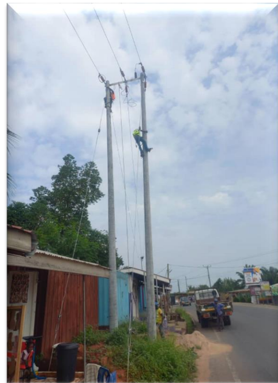
Stringing of 33KV Overhead line Nsawan – Aburi Road, March 2023
