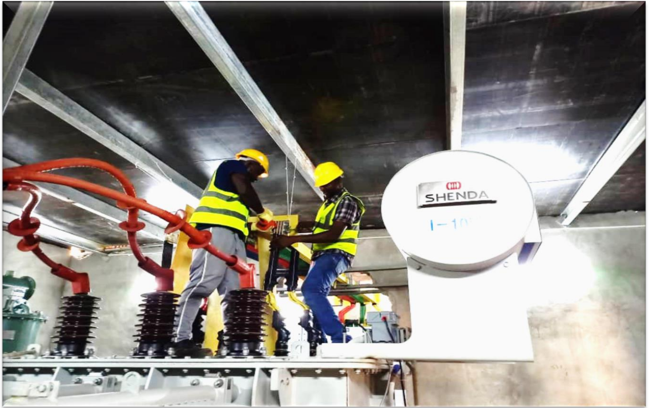
Newly Installed 4MVA Transformer by Gross Pool Engineering Team at Yunzu Fiber Factory, Near Nsawam E/R, Ghana January 2023
