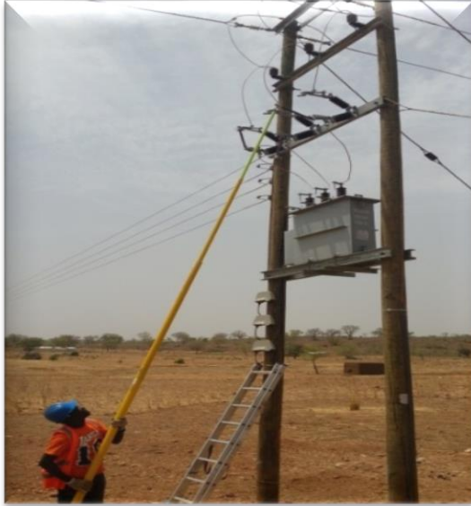
Commissioning of PMT substation at the Nabdam District in the Upper East Region of Ghana
