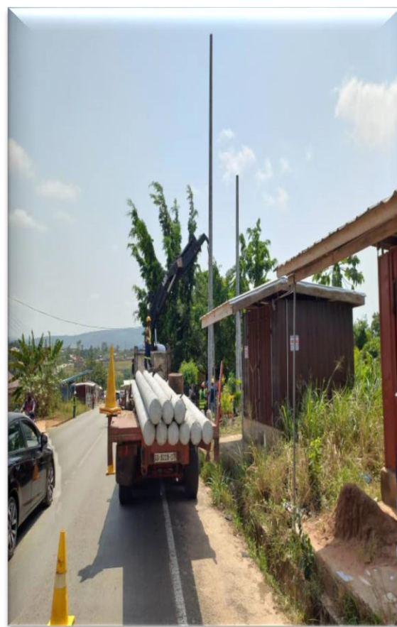
Planting of 15M Spun Concrete Pole for the Construction of 33KV Overhead / Underground line on the Nsawam – Aburi Road Feb. 2023
