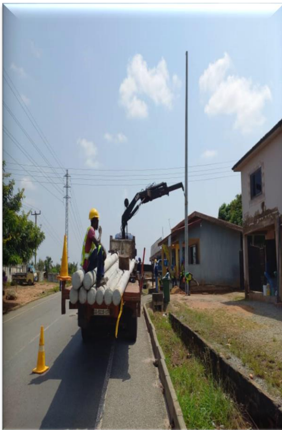
Planting of 15M Spun Concrete Pole for the Construction of 33KV Overhead / Underground line on the Nsawam – Aburi Road Feb. 2023
