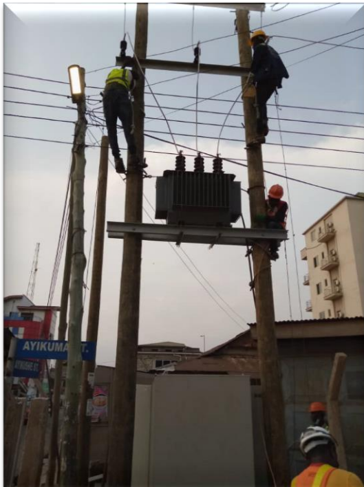
Mounting and Dressing of PMT Substation at Ashawo market, Adabraka – MiDA Project (Kaneshie District)
