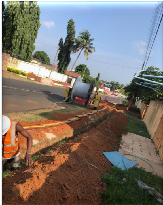
Laying of Under Ground Cable at SS Omane Street – MiDA Project (Kaneshie District)
