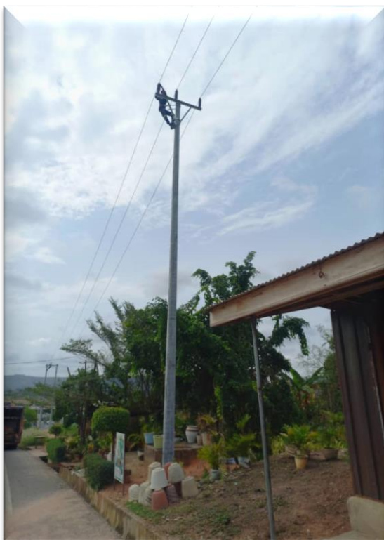
Stringing of 33KV Overhead line Nsawan – Aburi Road, March 2023
