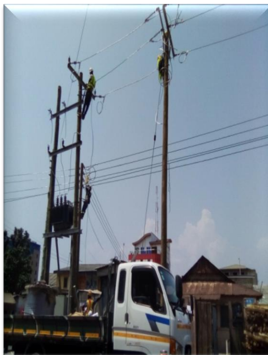
Mounting and Dressing of PMT Substation at Ashawo market, Adabraka – MiDA Project (Kaneshie District)
